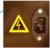
Charger connection point
